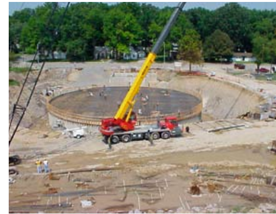
Construction of stormwater holding tank at McMillan Park as part of the Camp Scott Wetlands project. Photo: City of Fort Wayne Utilities.
